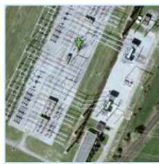
Pilot installation Nehden, DE 3rd party NCIT, REB500
