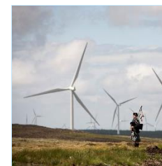
Real installation UK SAM600, FOCS 670series, 3rd party
