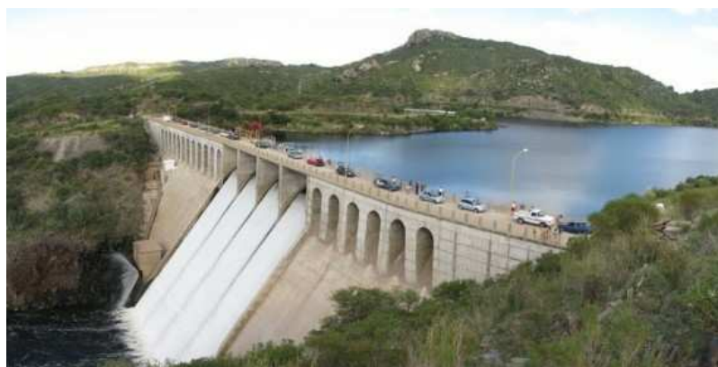
Figure 5: Dique La Huertita
